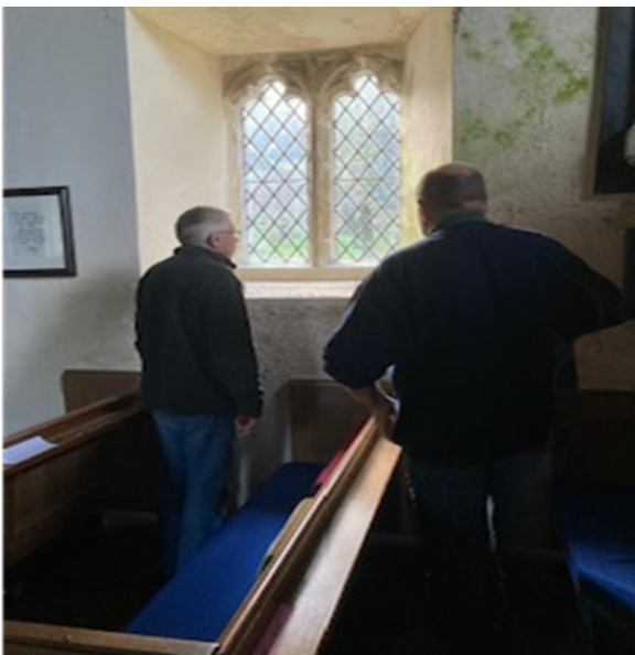
The bolts are uncovered!
